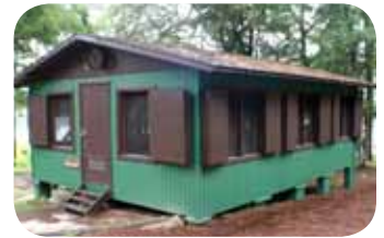
Many sponsors have already agreed to renovate cabins at Camp Winona.
